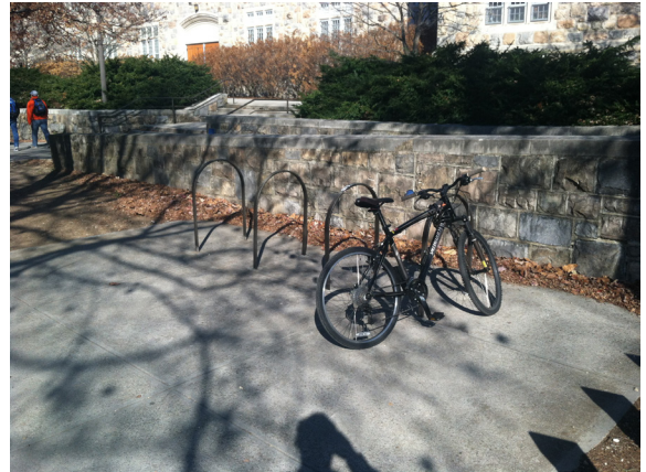
14: Two of four staples are loose. Recommend cut and repour concrete and remount to vertical.
