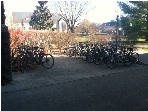
7: Half of racks are loose recommend immediate cut and repour concrete or replace with inverted-U rack.
