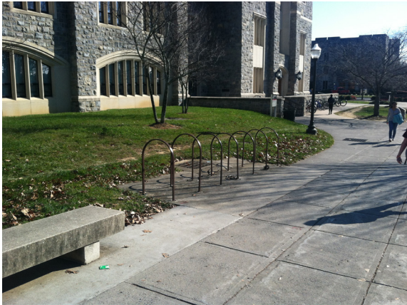
11: Two staple racks are loose, recommend cut and repour concrete.
