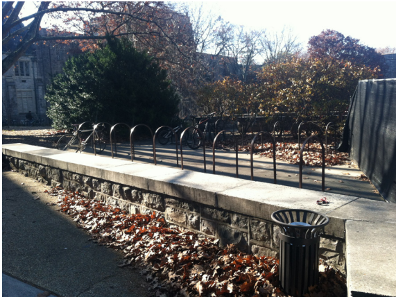
5: Almost all staples are loose, adjacent inverted-U is fine. Recommend cut and repour concrete or replace with new 10 rack inverted-U (2x5 rack).
