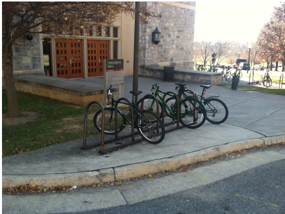
12: Existing Inverted-U rack was hit by a vehicle and if functional, but recommend replacement with new inverted-U if possible cut to salvage 4 of 5 units.
