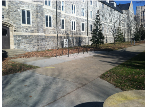
8: One staple is damaged, others are loose. Recommend removal of bent staple and cut and repour concrete on remaining.
