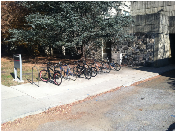
6: 11 staples at Slusher are in functional repair, most are minimally loose, repair needed in a few years.
