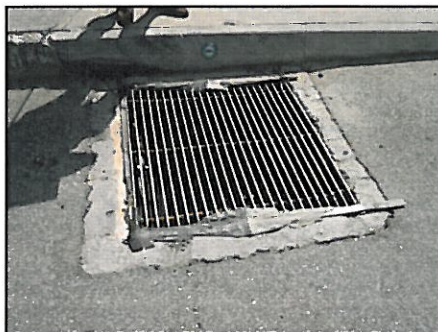
Drop Grate Inlet 8038
