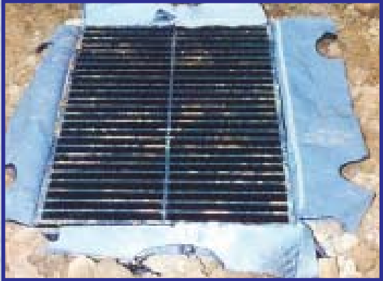
installed Siltsack held in place by grate.
