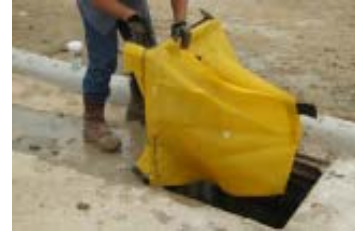
Slide Siltsack® over opposite side of grate.
