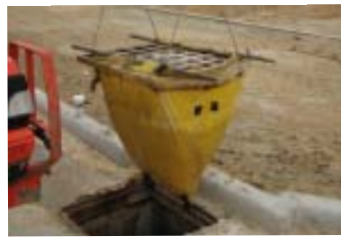
Removed Siltsack® is now ready for cleanout.
