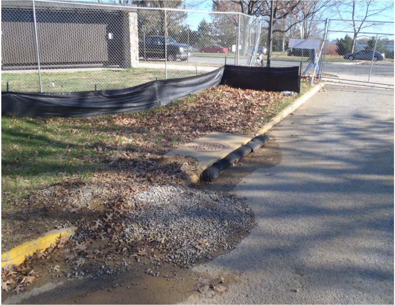
Rapid Flow Curb Inlet Protection with Polystyrene Aggregate
