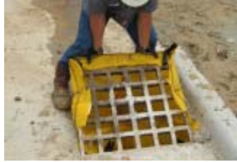
Slide Siltsack® over one side of grate.
