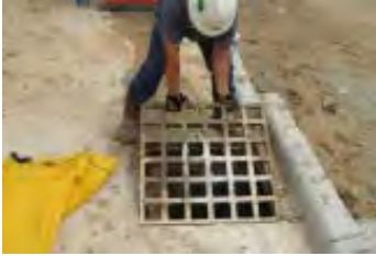
Remove grate from catch basin.
