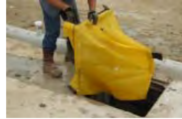
Slide Siltsack® over opposite side of grate.
