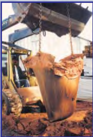
Sediment captured by Siltsack® can easily be removed from the site.
