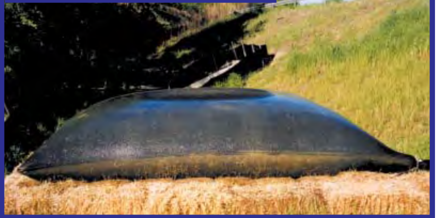
Hillside Installation on Straw Underlayment
