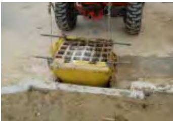
Slowly remove Siltsack® from inlet.
