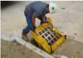
Replace Siltsack® and grate inlet into recess.
