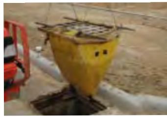
Removed Siltsack® is now ready for cleanout.
