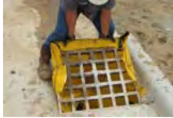
Slide Siltsack® over one side of grate.
