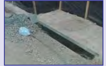
Failed Inlet Protection
