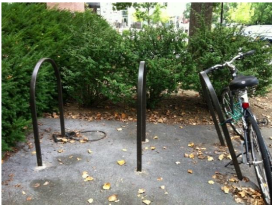
Staple Racks at Randolph Hall in need of repair
