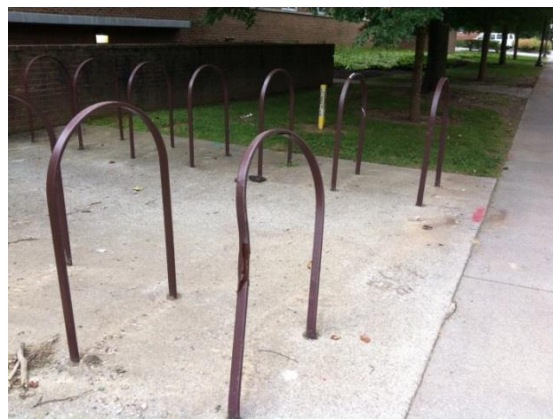
Damaged Staple Racks in the Upper Quad
